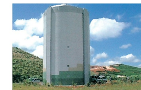
Hiraodai Distribution Reservoir
