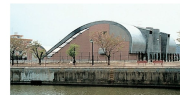
Kinzangawa Pump Station
