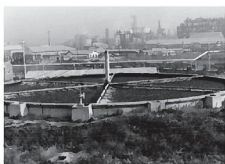
Trickling filter of Kogasaki Sewage Treatment Plant
