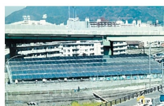
Murasaki River Solar Power Plant
