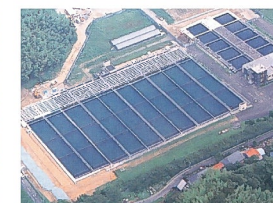
Ideura Water Purification Plant (Completed in 1972)
