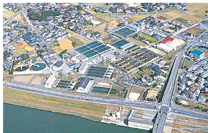
Isaza Intake Treatment Plant (completed in 1944)
