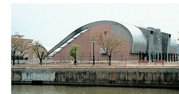
Kinzangawa Pump Station
