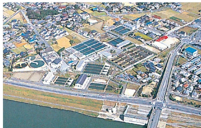
Isaza Intake Treatment Plant (completed in 1944)
