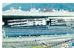
Murasaki River Solar Power Plant
